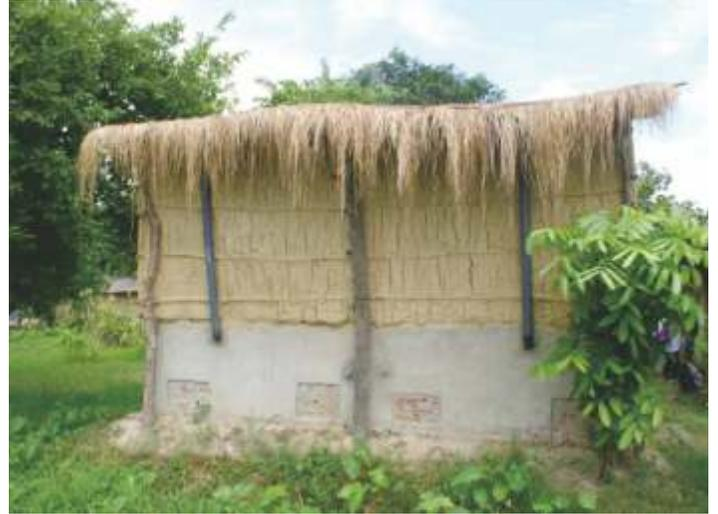
Figure 3. Soil is compacted to build a hill on which the UDDT is constructed
