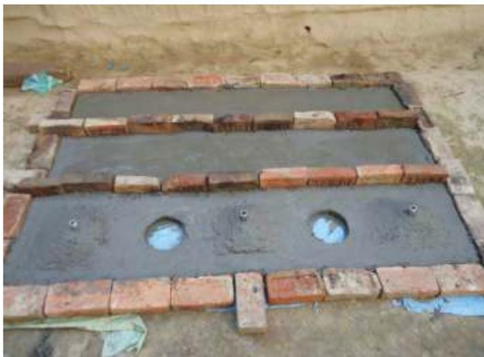
Note: A completely rectangular toilet top can be used when the superstructure is built with bricks.
