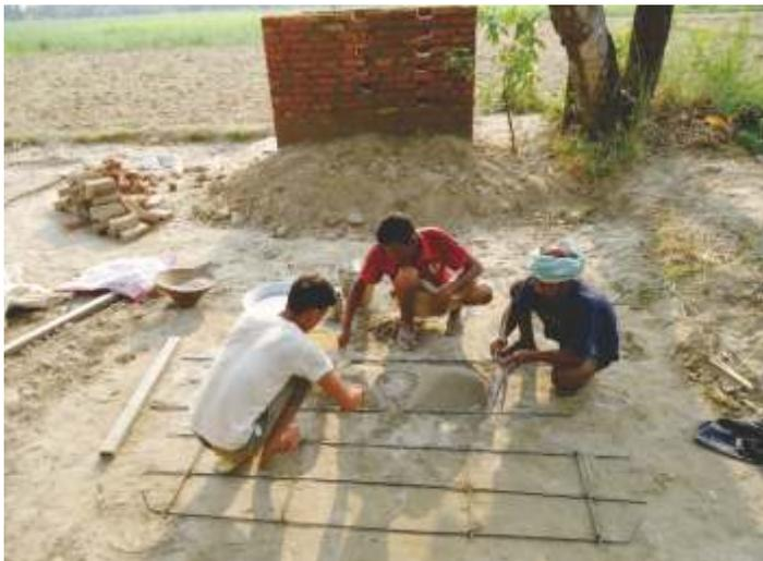
Figure 11. Preparing the casting mould
