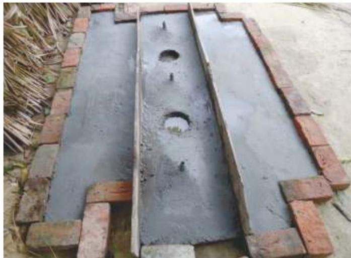
Note: The side elements of this top element have right-angled edges in all four corners that allow the fitting of bamboo poles for a semi-permanent superstructure with woven mat walls.
