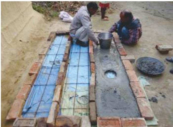
**Figure 13. Drying pre-cast elements in the casting mould**
