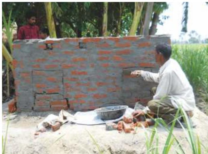
Note: Mason marks where the collection chambers will be opened once faeces are decomposed. Future openings are not cemented permanently but closed with bricks and local mortar to withstand flash floods.
