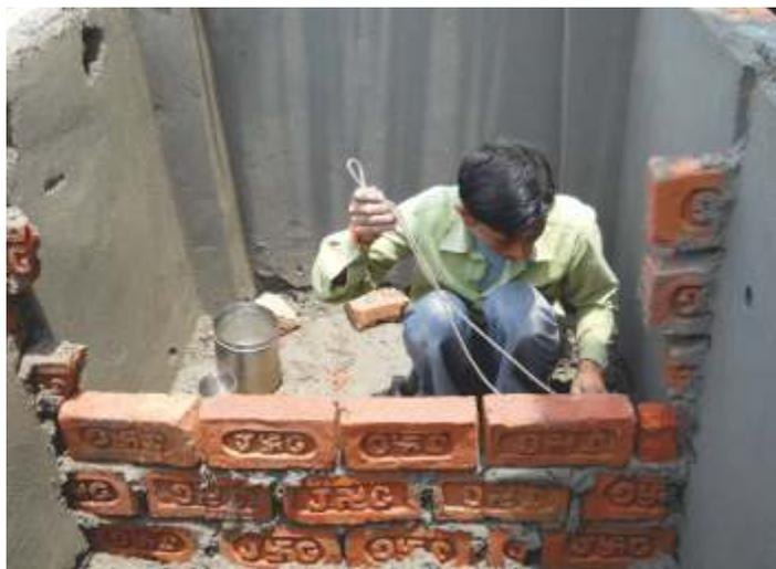
Note: Walls and ground are cemented from inside as well as outside. The wall inside the substructure separates the two collection chambers. The hole on the left upper corner holds the ventilation pipe.
