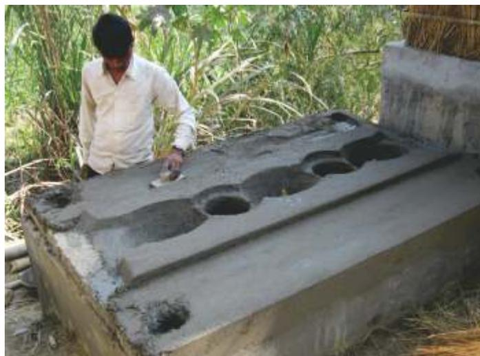
Note: The squatting pan was put on top of the substructure and is being fixed and plastered.
