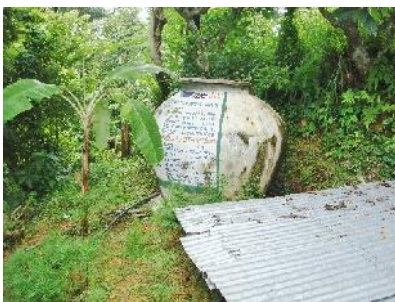
1. Multiple Water Use System collection tank
